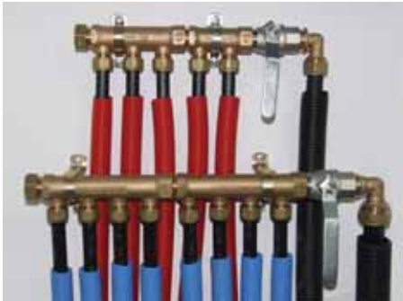
Hot and Cold Distributors installation - general view
