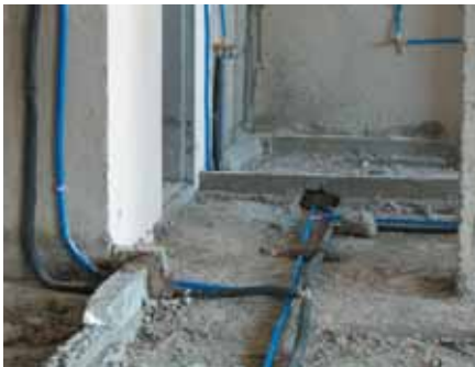
Concealed Installation before covering and flooring
