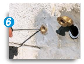
Attaching the 105° elbow to the plastic box After connecting the 105° elbow to the PEXGOL pipe, push the extra length of pipe back into the conduit pipe by pushing the plastic box in the direction of the
